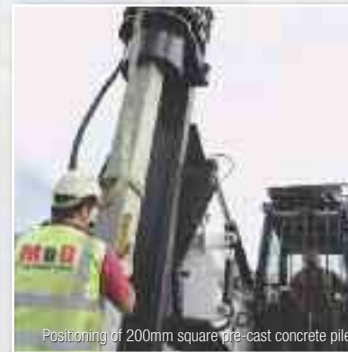
Installation of 200mm square pre-cast concrete pile
