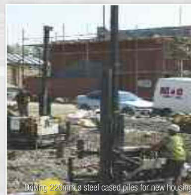
Driving 220mm \phi steel cased piles for new housing
