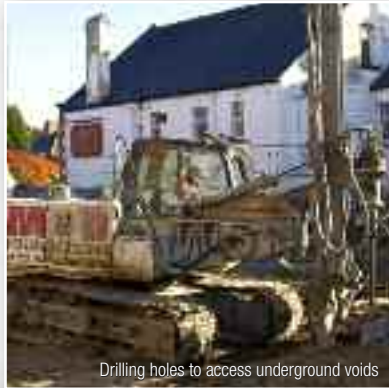
Drilling holes to access underground voids
