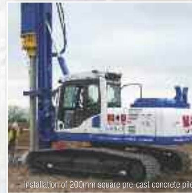
Installation of 200mm square pre-cast concrete pile
