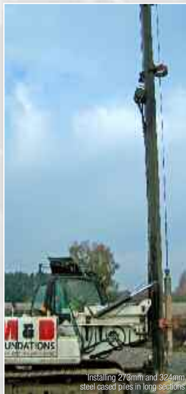
Driving 220mm \phi steel cased piles for new housing
