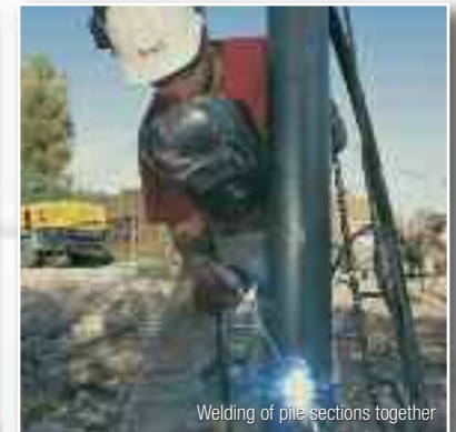
Welding of pile sections together
