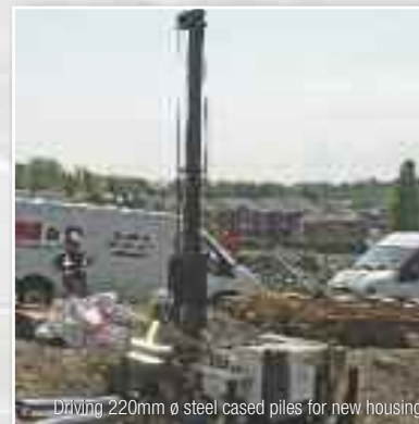
Driving 220mm \phi steel cased piles for new housing
